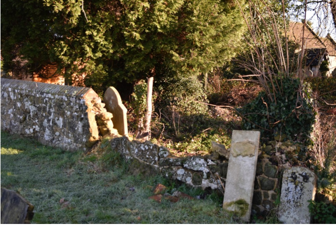
BEFORE: Needing urgent repairs
